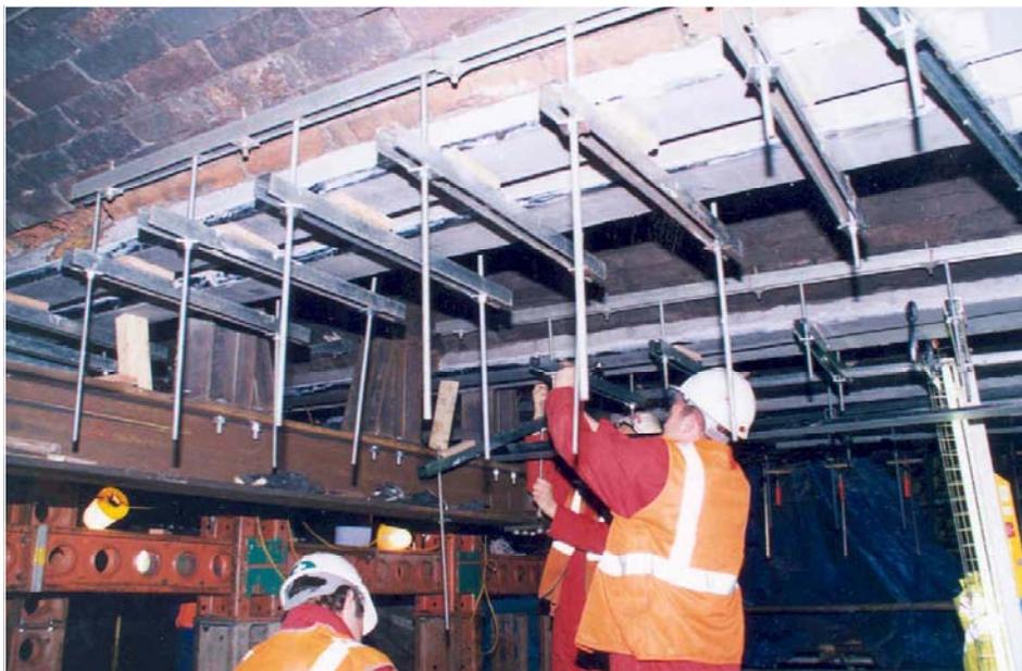
Installation was completed strictly in accordance with the method statement. After the surface preparation was inspected, a thin layer of epoxy adhesive was applied to the beam by trowel, ensuring full wetting of the surface and that all local pitting was filled. A peaked layer of adhesive was applied to the laminates, thicker in the middle than at the edges, so that as the laminates were pressed into place air would be expelled and not trapped within the bond line.
